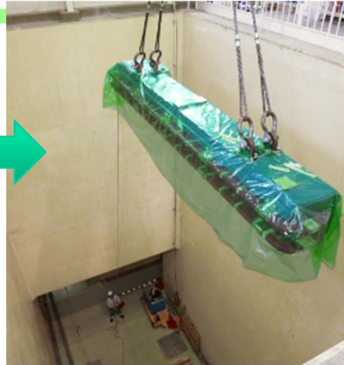
move into tunnel
