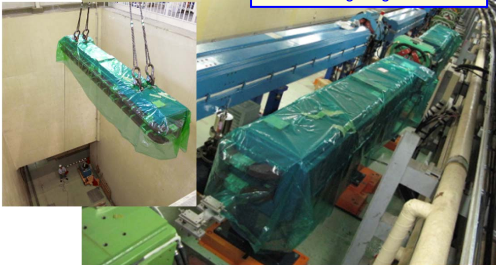
Installation of 100 new long LER bending magnets done
