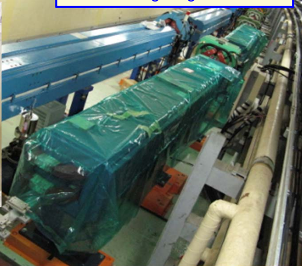
Installation of 100 new long LER bending magnets done
