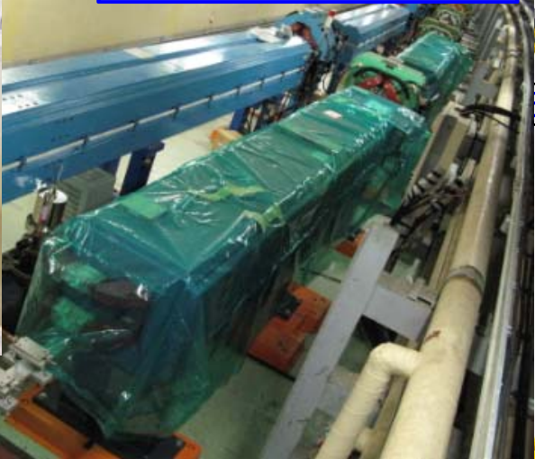
Installation of 100 new long LER bending magnets
