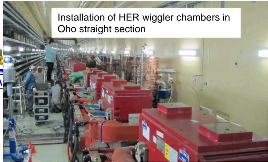
Installation of HER wiggler chambers in Oho straight section
