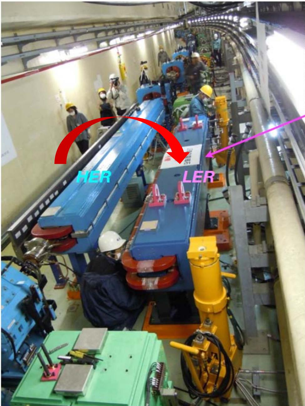
All 100 4 m long dipole magnets have been successfully installed in the low energy ring (LER)!
